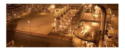
Port Said NGL Plant has been designed for deep extraction of NGL cut from a mixed feed gas; it is classified as one of the largest NGL plants in Egypt regarding the plant processing capacity reaching about 1350 million standard cubic foot per day (MMSCFD).
